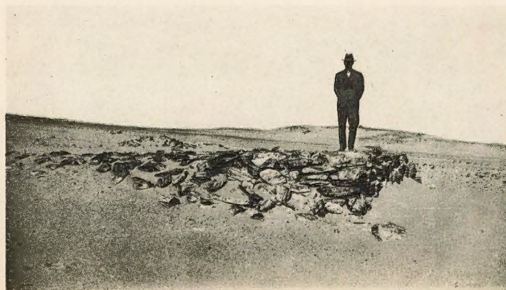
3. - Ramp of diorite-gneiss for loading blocks. S. area.
